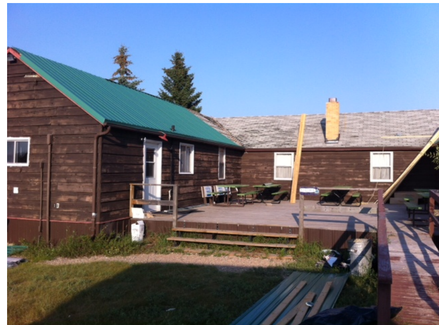
Baden Powell Lodge – August 2012 as new roof is being installed
